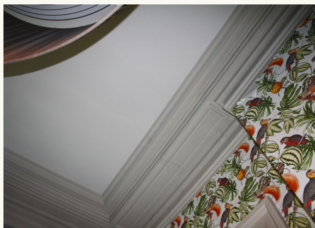
scheuren in molures
